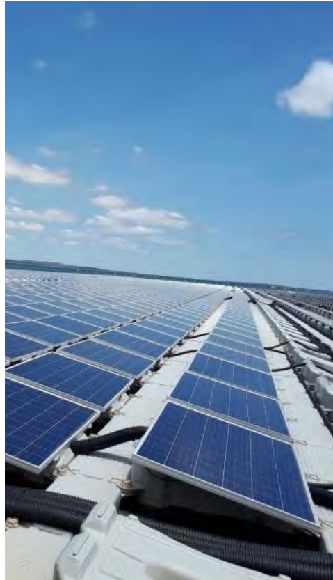
This floating photovoltaic power plant in Bahia, Brazil is filled with 2,500 liters of FR3® insulating vegetable oil and has the capacity to generate one megawatt-peak (MWp) of energy.
